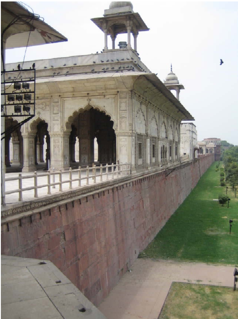
Plate 9.7: Eastern edge of the Fort seen from the Ring road, a significant view; CRCI 2006
